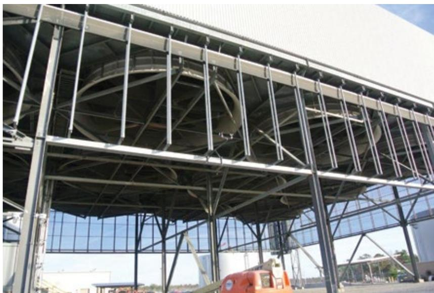
14. Caithness screens are shown retracted (front) and deployed (right side and rear)
