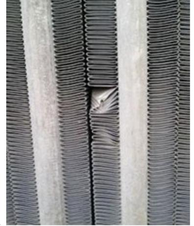
**19, 20. Achieving maximum performance** involves thorough inspection and the plugging of the smallest leaks with red gasket-forming silicone (above) and monitoring of fin condition and continually repairing damaged areas (right)
